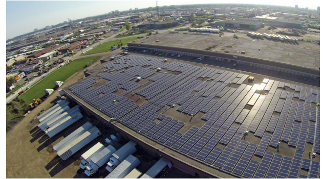
600 kW DC FIT 2 Project located in Brampton, Ontario.
